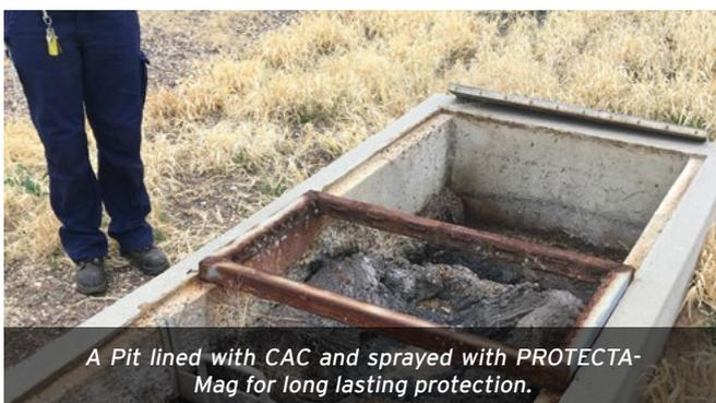
A Pit lined with CAC and sprayed with PROTECTA-Mag for long lasting protection.
